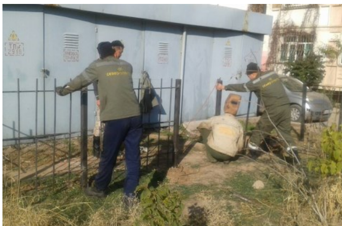
Constructing fencing the electricity power transformer in Kok-Zhar, Kyrgyzstan (Credit: NDI)
