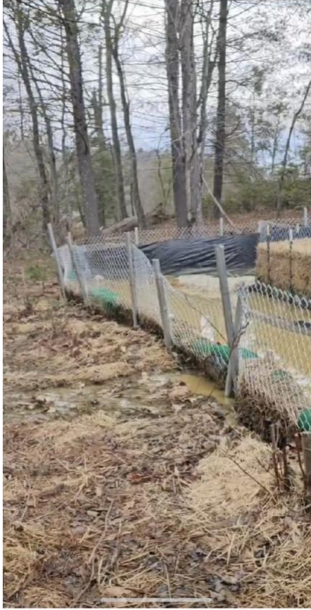
Left, Figure 9 - sediment trap on MVP site discharging polluting water; Right, Figure 10 - Bottom Creek with sediment-filled flow channel downstream from the MVP work site. January 12, 2024
