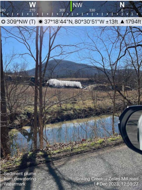
Figure 7 - A view of Sinking Creek, more than six weeks prior to the photos above, showing pollution entering the stream from MVP sites upgradient. Volunteers first found the cloud of turbid water from sediment basins hugging the stream bank and in sharp contrast with the clear stream flow. December 14, 2023.
