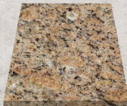
After Crack Repair
