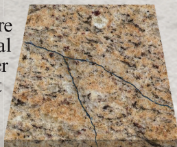
Before Crack Repair
