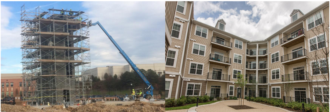
Oxford Square construction.
