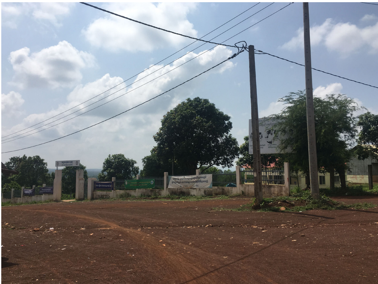
Access road into Prey Meas, showing the O' Clor health care center.
