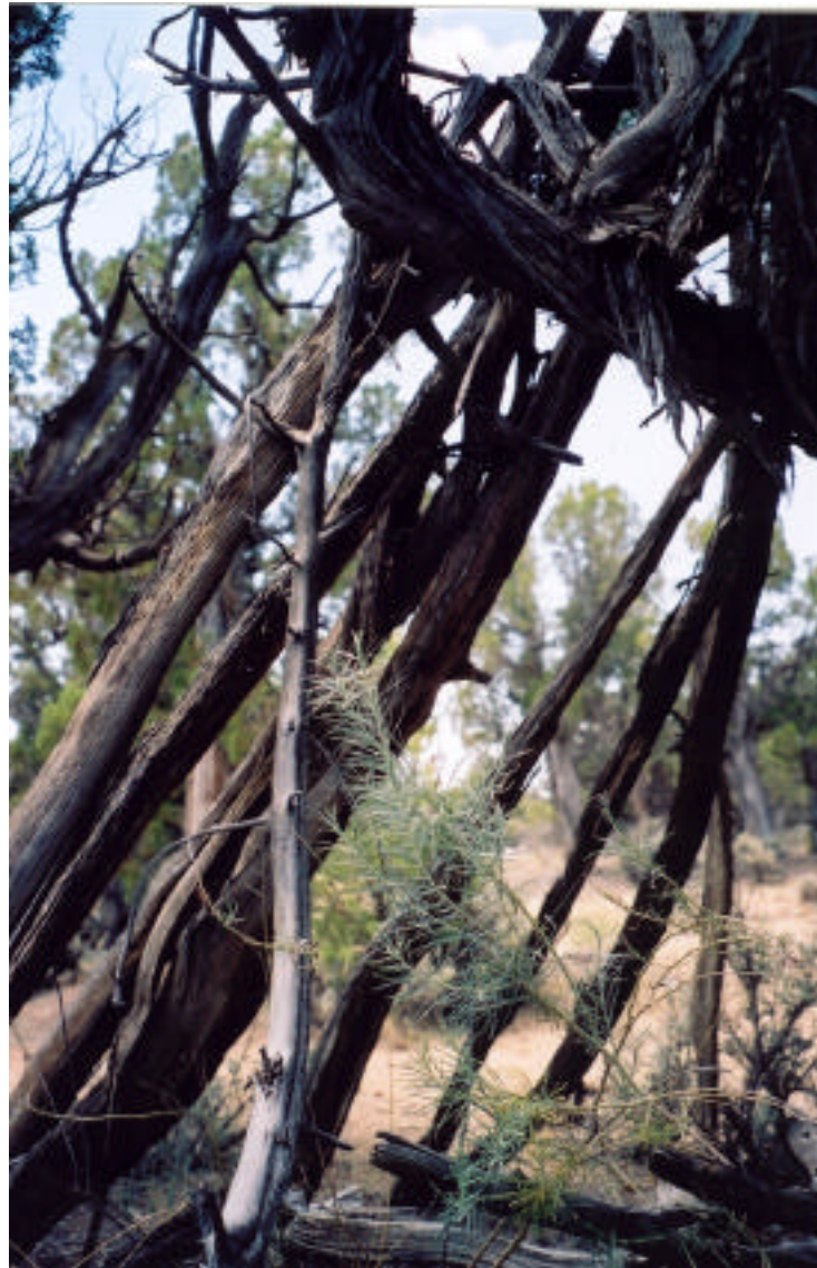
Plate 14: Example of a photograph showing the interior of a structure
